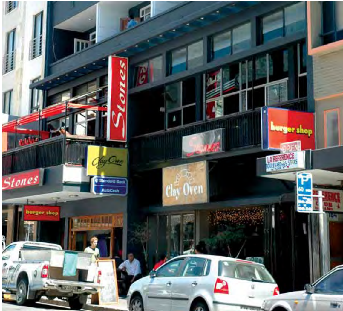
Figure 15: Mixed use building with residential accommodation above shops
