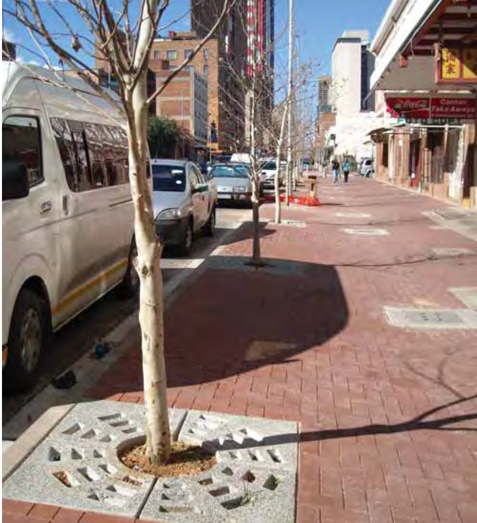
Figure 11: A Vibrant Pedestrian Route in Mitchells Plain Town Centre.
